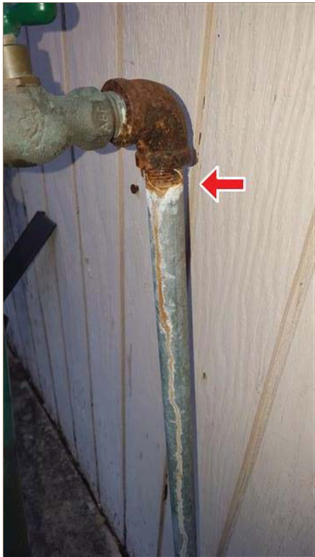
(6) Water intrusion at the main water entrance to the house. Piping should be insulated to keep from freezing in cold weather.
