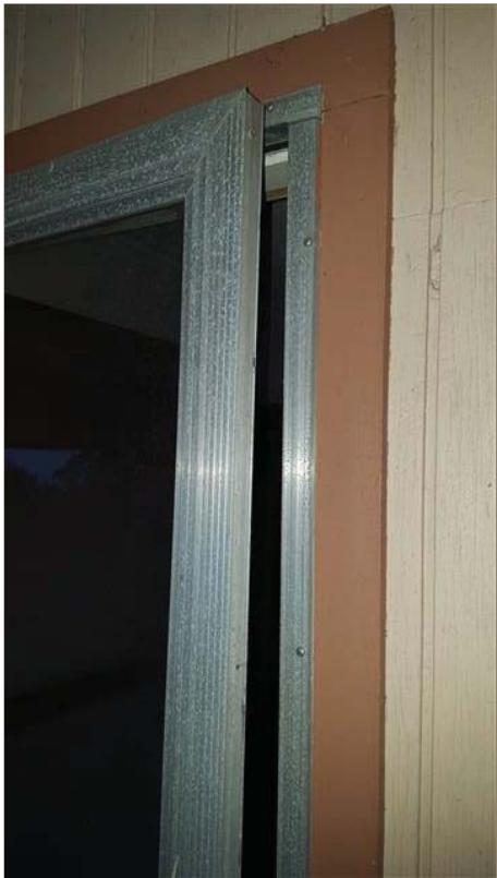
(2) Screen door at back porch is damaged.
