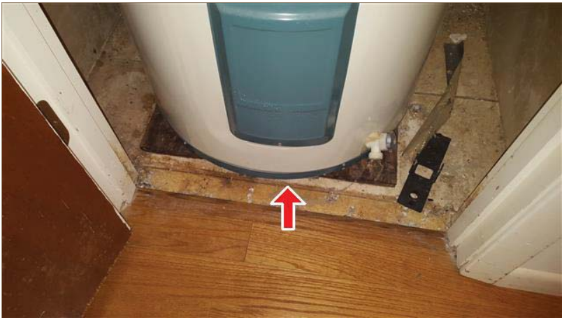
(2) Secondary drain pan missing from water heater.
