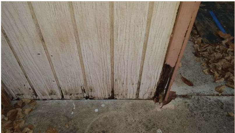
(3) Paint is peeling from exterior walls of the house.
