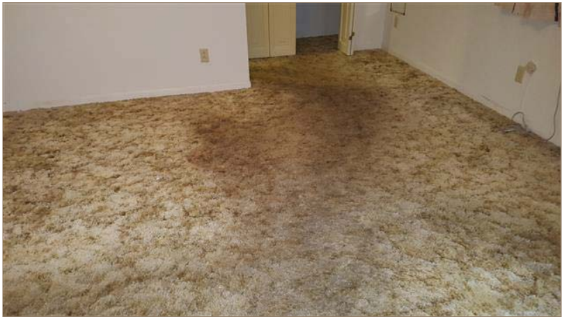
(3) Water damage to floor at garage addition near the sliding glass door.
