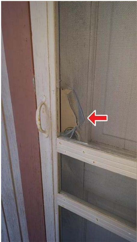
(2) Screen door at back porch is damaged.
