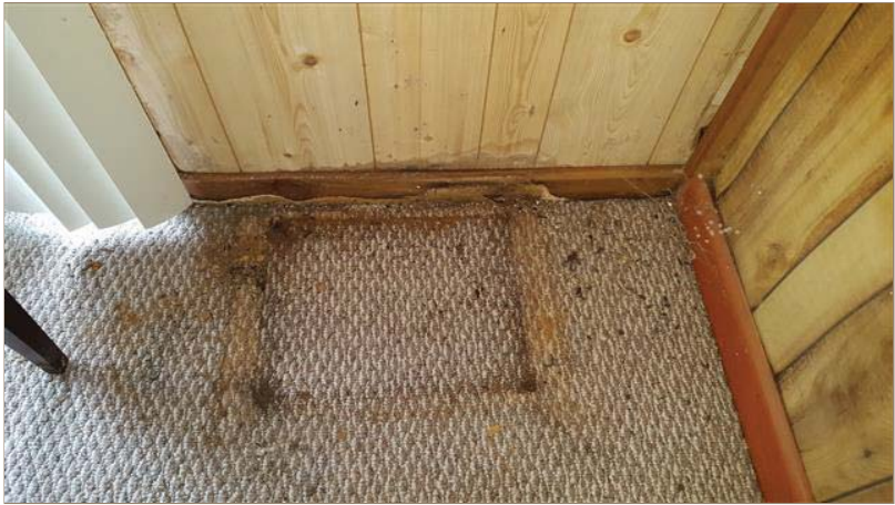
(3) Water damage to floor at garage addition near the sliding glass door.
